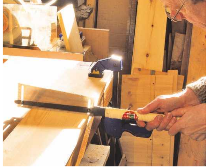
▲ Pic.2 Cutting shelf housings to depth
